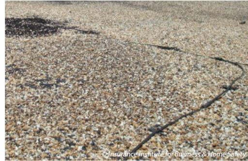
*Built-up roof cover with gravel embedded in asphalt. (A lightning protection cable also is shown.)*
