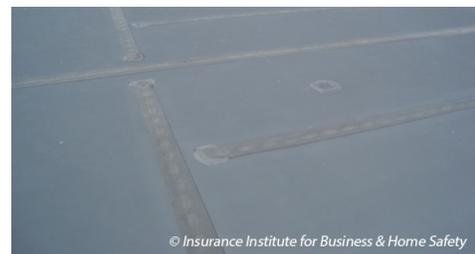
*Single-ply EPDM membrane roof cover (mechanically attached).*
